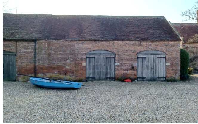
West Range Barn (East Elevation)
