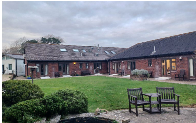
Existing IPU building
