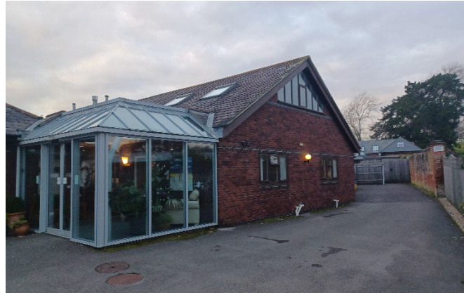
Existing IPU building
