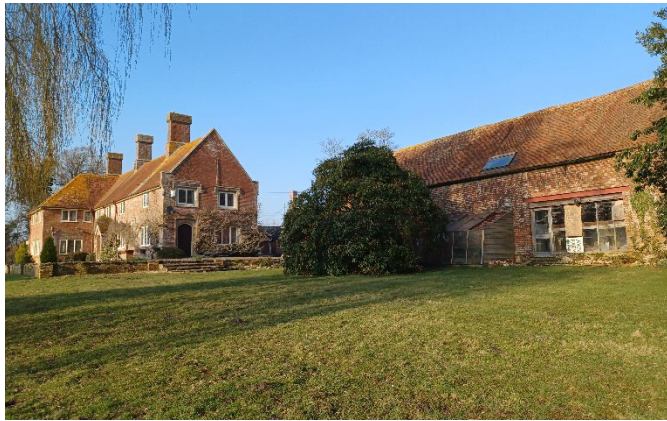
Rear view of severance
