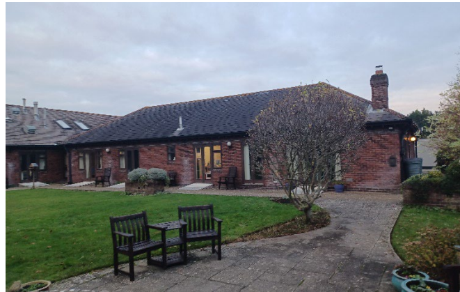
Existing IPU building
