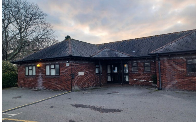
Existing IPU building
